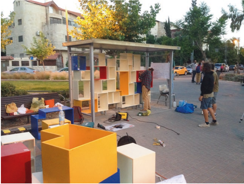
Fig. 6.4 Establishing the reading station in the German Colony. Photo: Eytan Shouker
